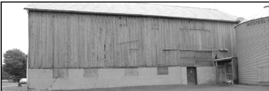
Prior to the foundation being added, the threshing floor was on the ground. The large barn doors are still visible on the right.
