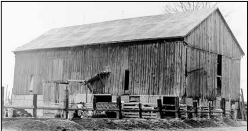
The threshing floor was on the ground. Srigleys added a foundation and made it all stable. A wooden silo inside the barn was torn out. Access to the upstairs was an outside ladder.
