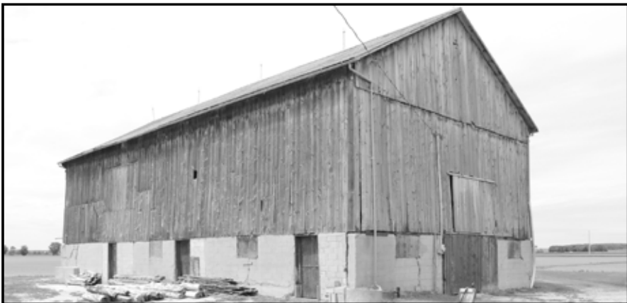
Prior to the foundation being added, the threshing floor was on the ground. The large barn doors are still visible on the right.
