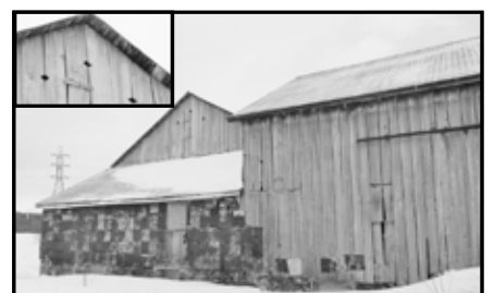
The barn at the back was smaller. The foundation was part stone, part cedar block. A ring was fastened into the stone foundation. The rest of the foundation had been cedar block.
