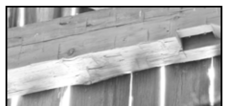
The sleepers were hand hewn on two sides, while the beams upstairs were hand hewn on all four sides.
