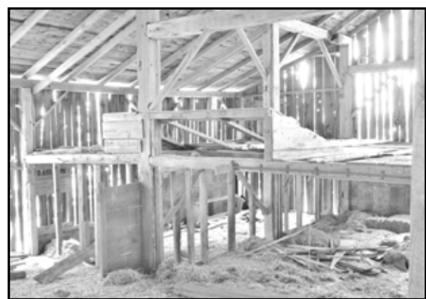
The boards have been removed from the granary, with the mow above. The threshing floor, with access up a gangway is to the left. A steel track is at the roof.
