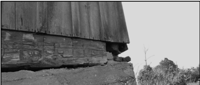
The barn was originally on mud sills. The single boarded stable was very cold, allowing in wind, rain and snow. Fred Priest helped raise the barn 7-8’ onto a cement foundation using railway ties to jack it up.
