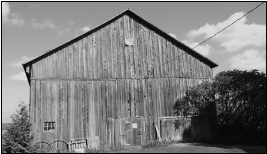
This bank barn was built into the side of a hill, with access to the threshing floor at ground level.
