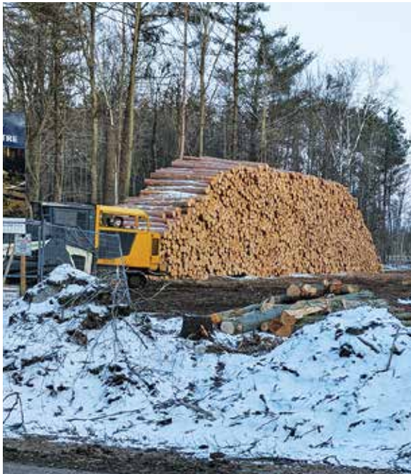
Photo courtesy of Mike Knell, Progress at Tiny Administrative Building
