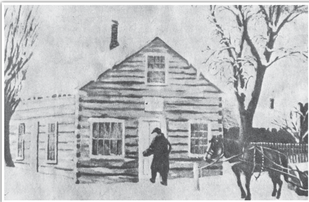
Elmvale's first post office building, on the corner of Queen and Yonge, built in 1863 and demolished in 1899. This is from a painting but the original painting has not been found. A photograph was taken just before demolition, but it also has not been found.
